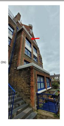
Protruding building at ground level has glass roof so simple access tower is not possible, approximate height of header is 8m.
